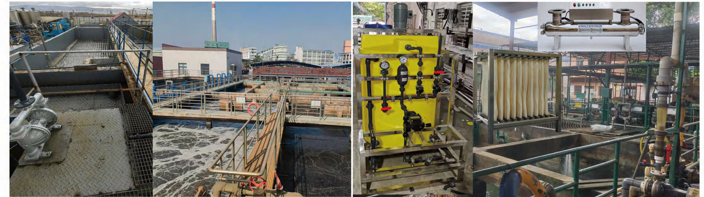
Food Wastewater Treatment Plant
